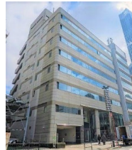
KM Shinjuku Building
